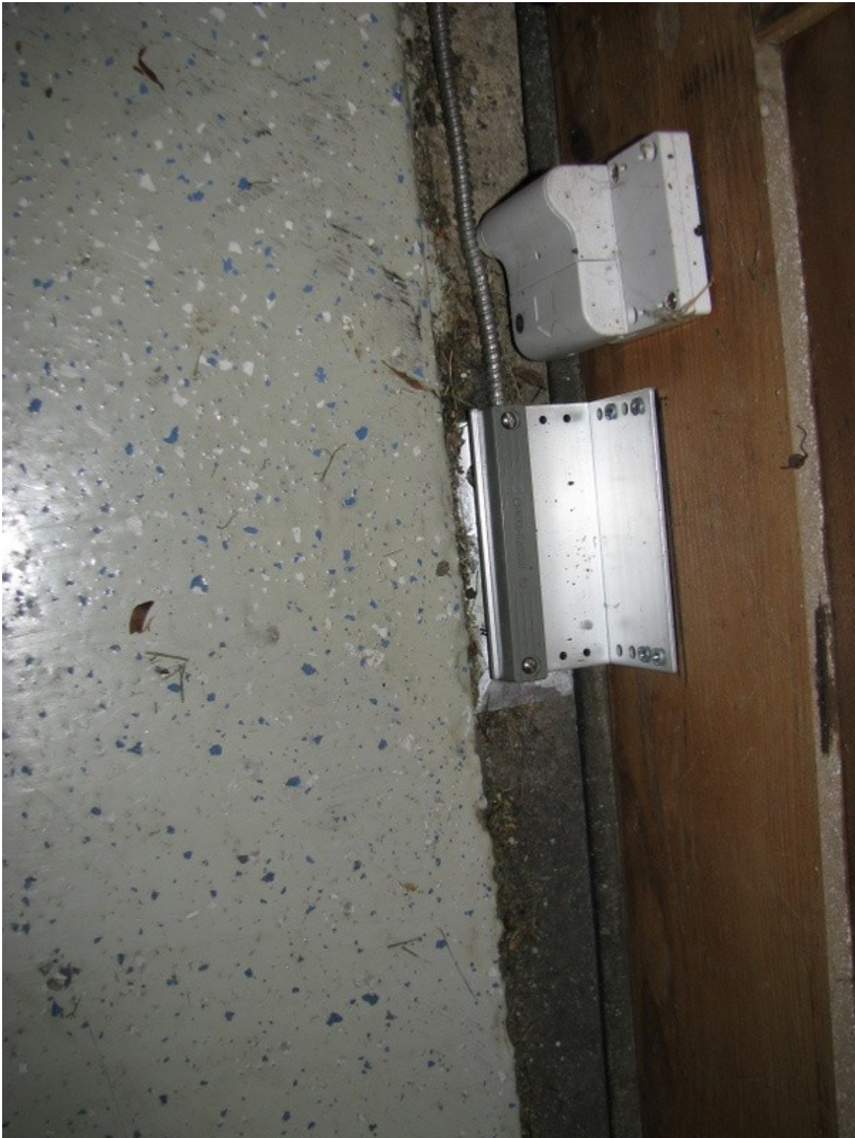
Industrial magnetic close limit switch to garage door controller.
